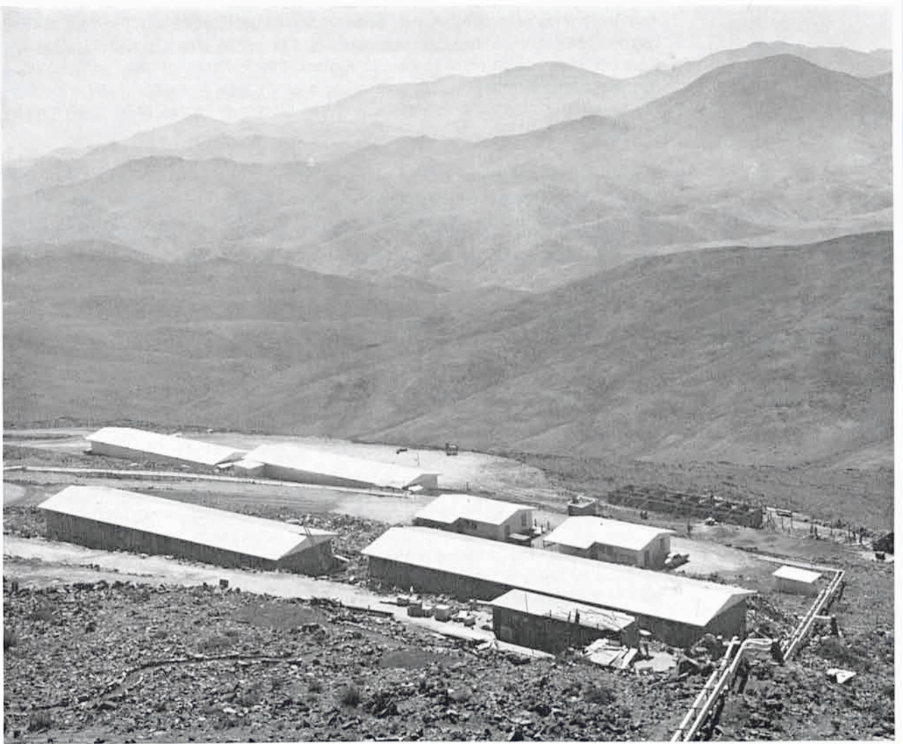
Construction project dormitories for technical staff, night assistants and astronomers.
