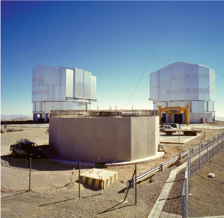
The foundation for the VLT Survey Telescope (VST) enclosure.
