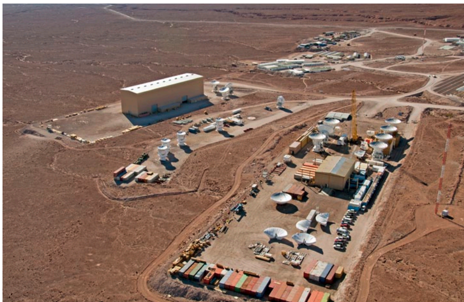
Aerial view of the OSF at 2900 metres altitude. In the foreground is the European antenna integration site with seven complete AEM antennas.
