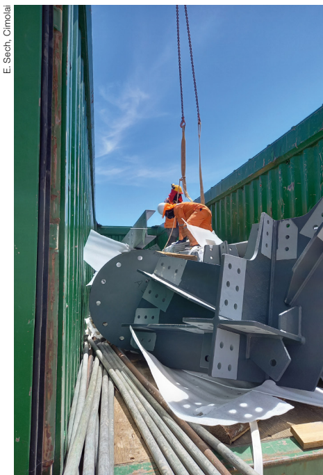
Container unloading at Cerro Armazones, ELT construction site.
