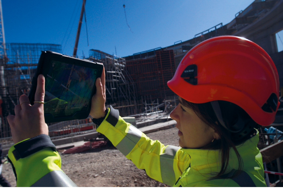
A worker on the ELT construction site holds a tablet computer, used for an augmented reality system that assists with the installation of components for the ELT's dome and main structure.
