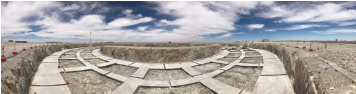
Panoramic view of the excavation for the auxiliary building which will surround the dome.
