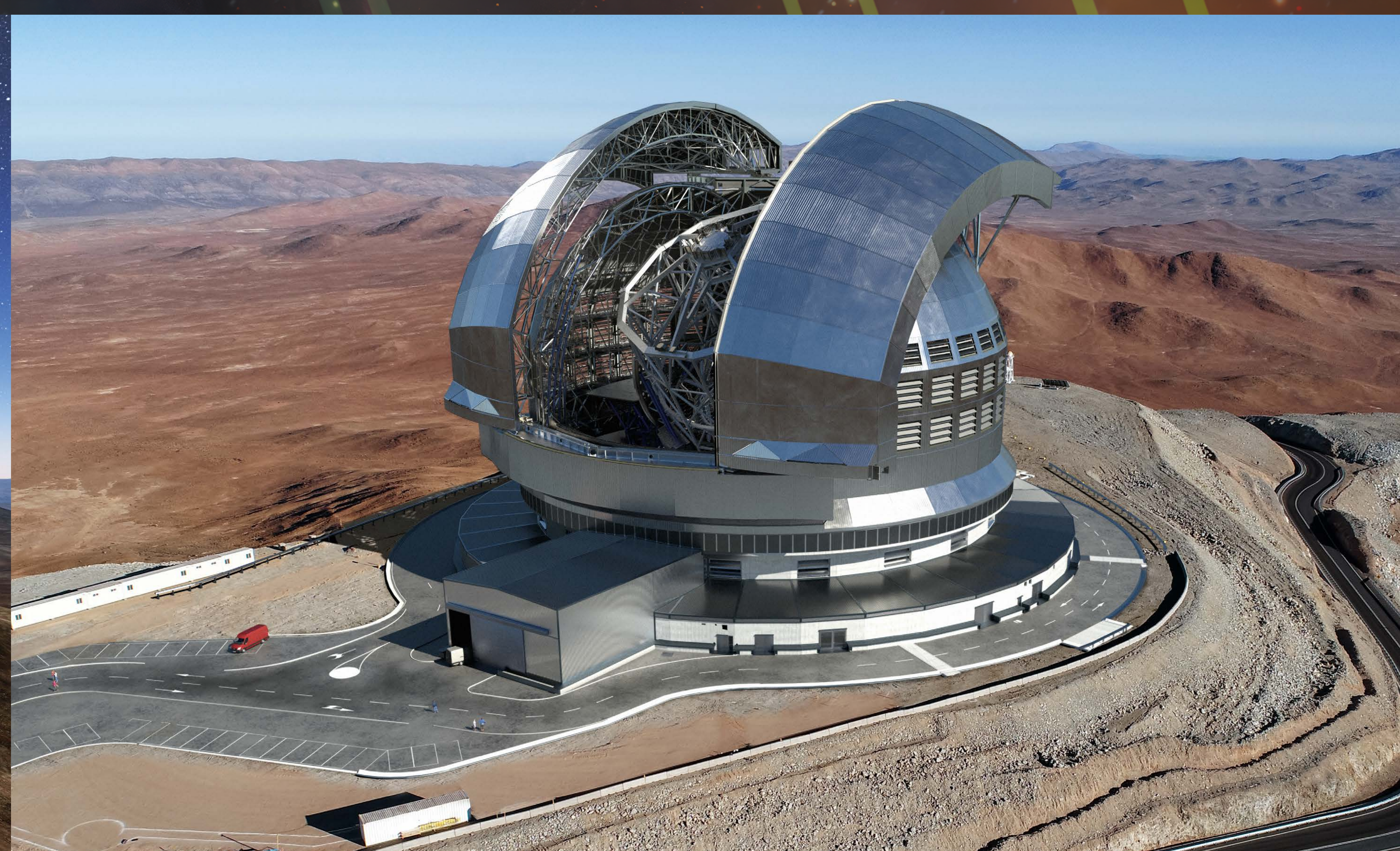
The sensitive and delicate components of the most sophisticated telescope ground-based astronomy has ever seen require special protection. This is especially true in the rough desert environment, with potentially damaging sand and wind, and in a country that is prone to earthquakes. The 80-metre-tall dome will shelter the ELT in windy conditions during observations and protect it and its delicate optics from the elements during the day. The dome is equipped with more than 100 seismic isolators to dampen earthquake vibrations.
