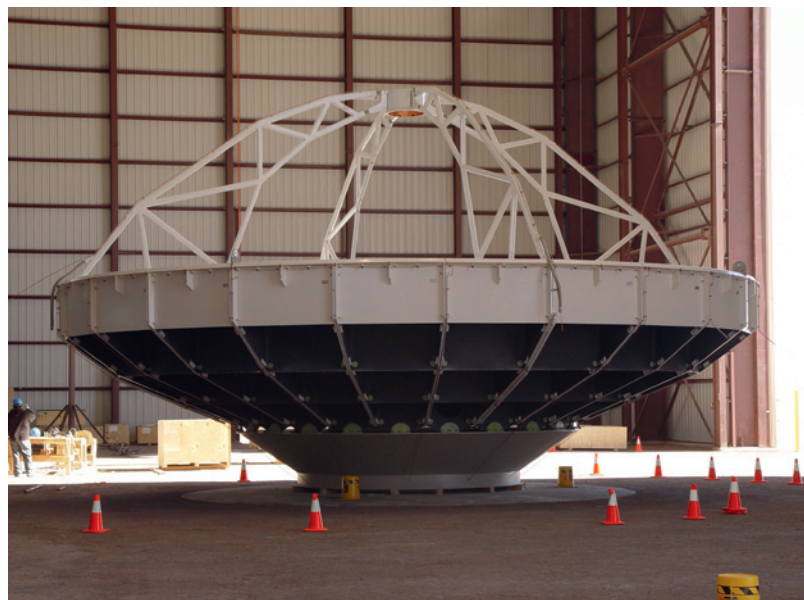
Figure 3 (left): The pedestal of the VertexRSI Antenna #2 in assembly at the OSF (Courtesy NRAO/VertexRSI).
