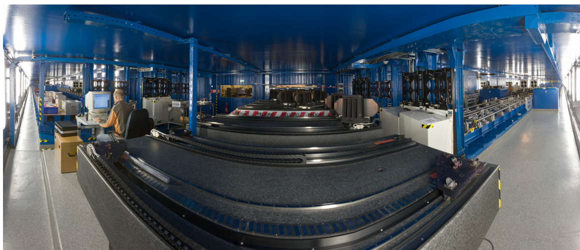
Panoramic view of the Very Large Telescope Interferometer (VLTI) tunnel, showing two delay lines.
