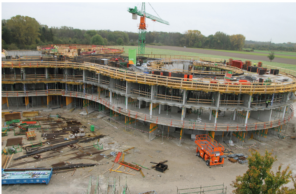
Construction of the extension to ESO Headquarters was begun at the beginning of this year and has now reached the second floor, as shown in this recent image. More details of the building concept can be found in a Messenger article (135, p. 2) and in Release eso1215.
