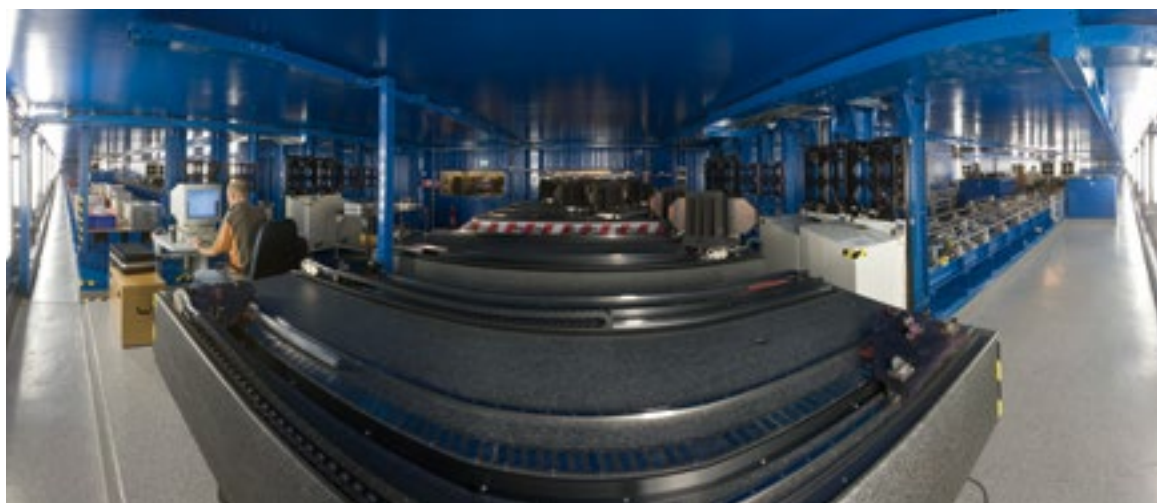
Panoramic view of the Very Large Telescope Interferometer (VLTI) tunnel, showing two delay lines.
