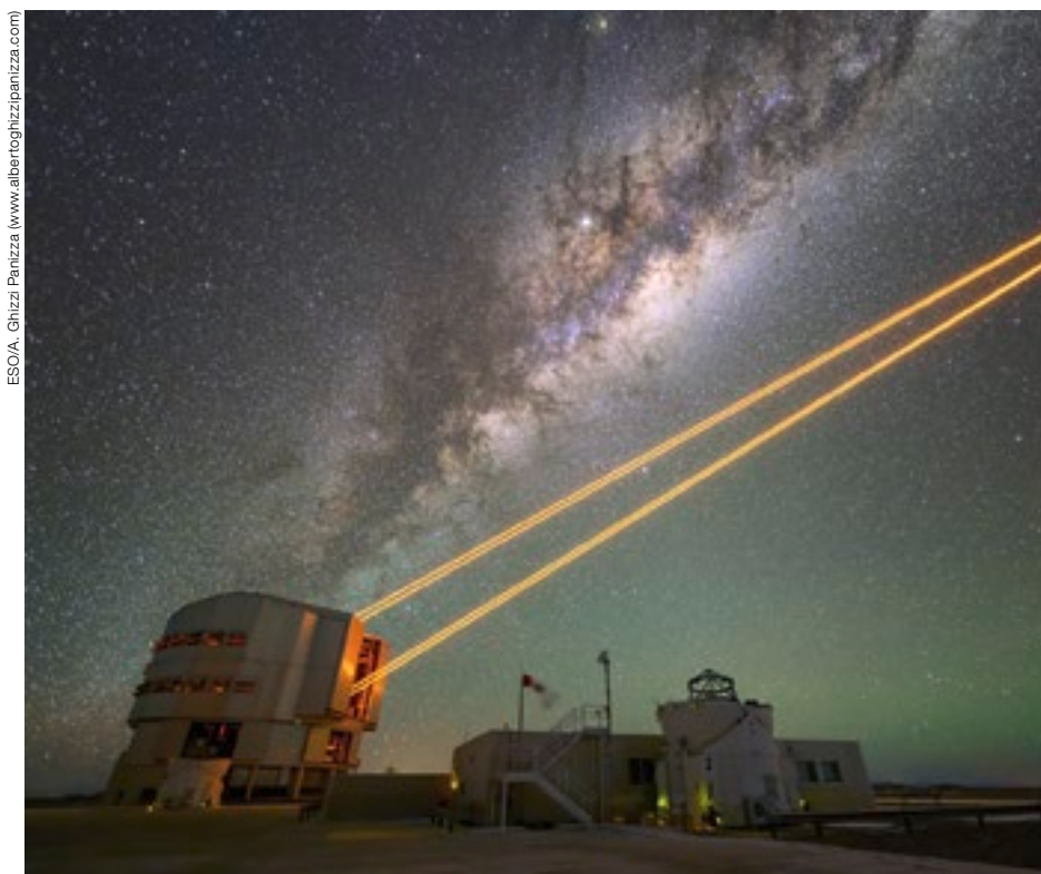
This picture of the week shows four powerful laser beams leaving Unit Telescope 4, or “Yepun”, at ESO’s Very Large Telescope (VLT) in Chile’s Atacama desert. These form the VLT’s 4 Laser Guide Star Facility, which enables astronomers to take extremely crisp images of the cosmos by employing a technology known as adaptive optics.
