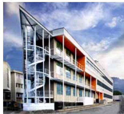
The building of the Partnership for Structural Biology, a joint activity of EMBL, ESRF and ILL
