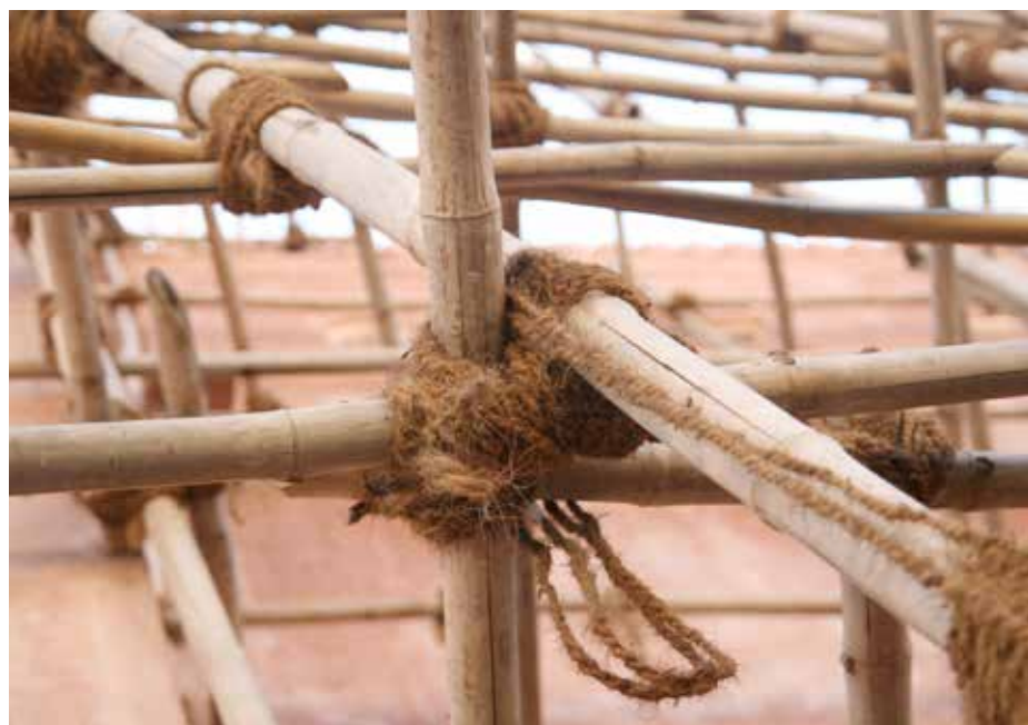
Rope-tied joints in traditional bamboo scaffolding
